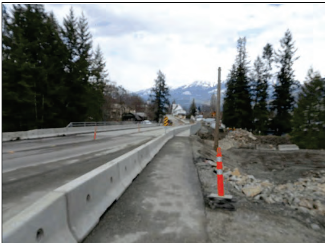
HIGHWAY 31/BRIDGE NE
