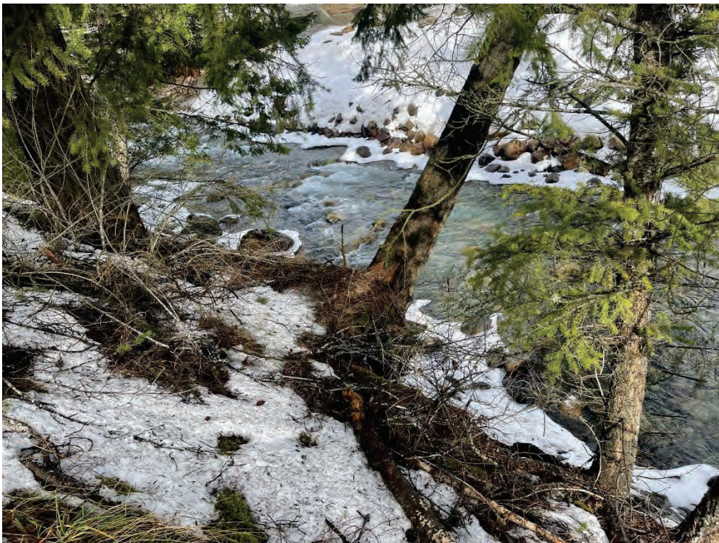
Photo 2: View of right bank erosion near site entrance off 3 rd Street
