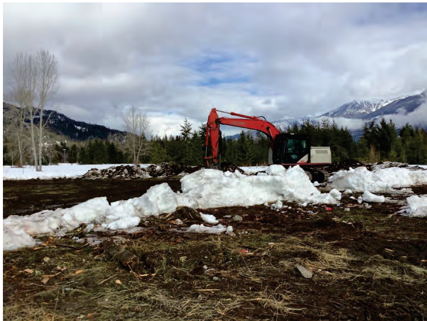
Photo 12. View of proposed development area looking northeast (Photo taken February 16, 2022).
