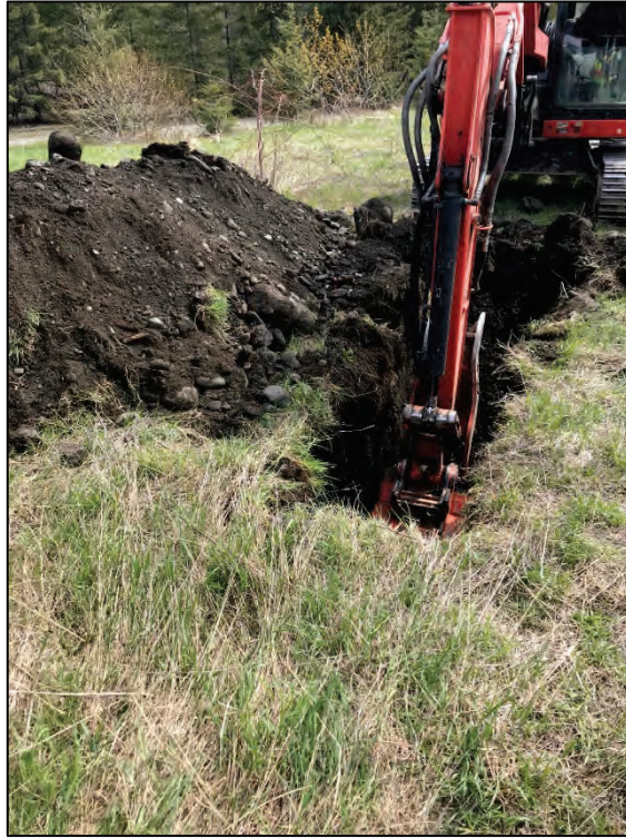
Photo 1: Looking to the northwest- digging APEC 3
