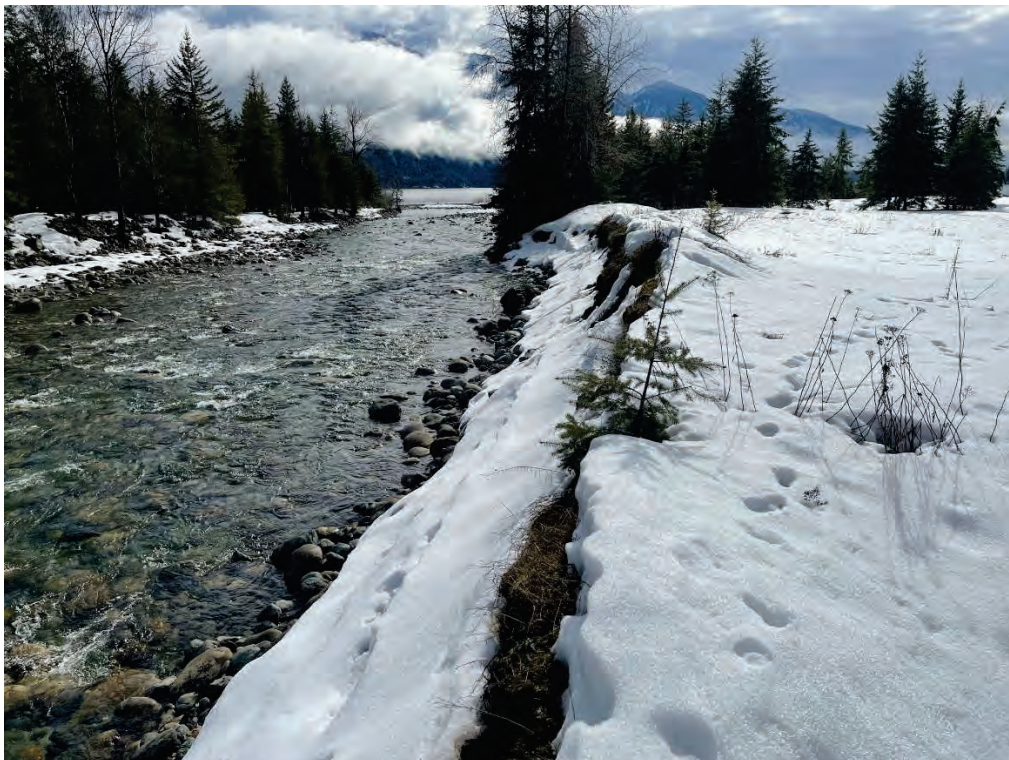
Photo 4: Looking downstream at right bank erosion
