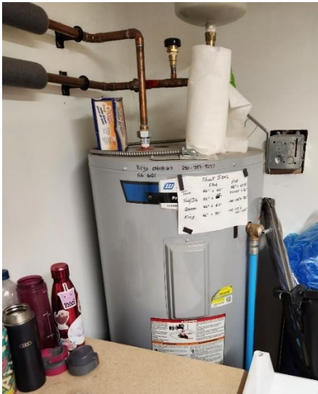
Figure 4 Electric DHWT
