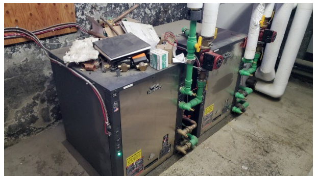
Geo-exchange heat pumps
