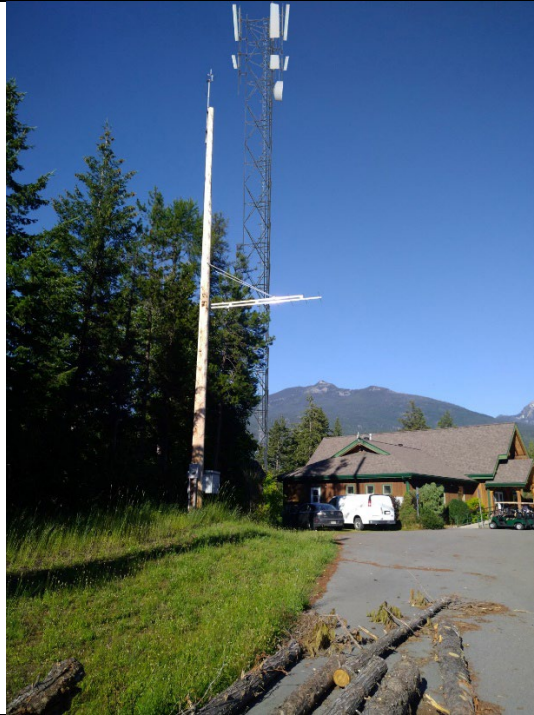
View: Looking east at tower from 5 th Street at the Kaslo Golf Club
