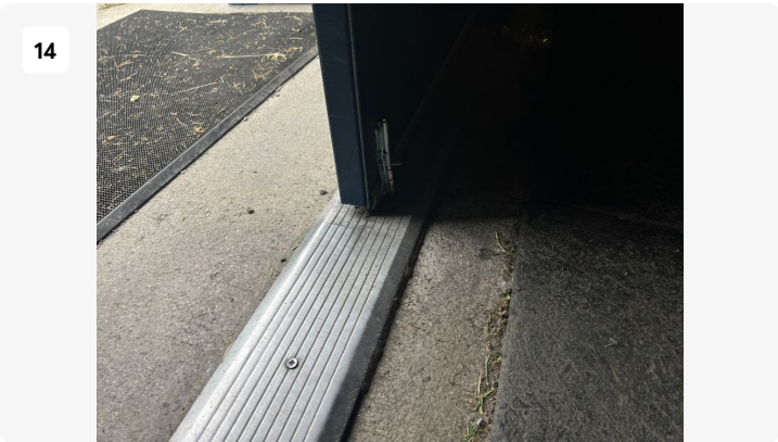
Change Room Entry Door 1. First threshold meets accessibility requirements.
