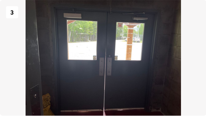
Main Entry Vestibule 1. No push buttons/auto door operators. 2. Door threshold appears to meet code requirements.
