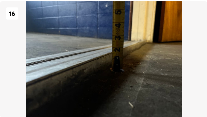
Change Room Entry Interior Door 1. Threshold does not meet accessibility requirements.
