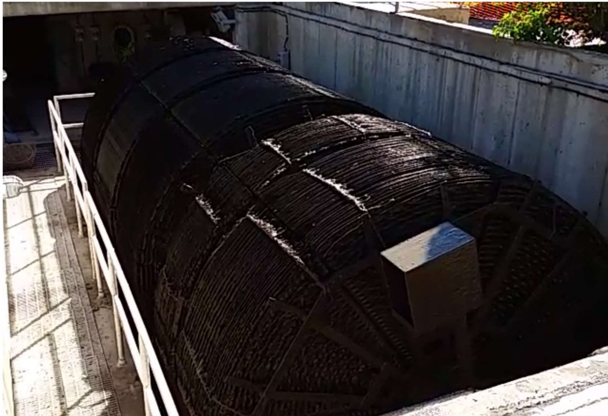
FIGURE 3-1: ROTATING BIOLOGICAL CONTACTOR IMMEDIATELY PRIOR TO REPLACEMENT IN 2017
