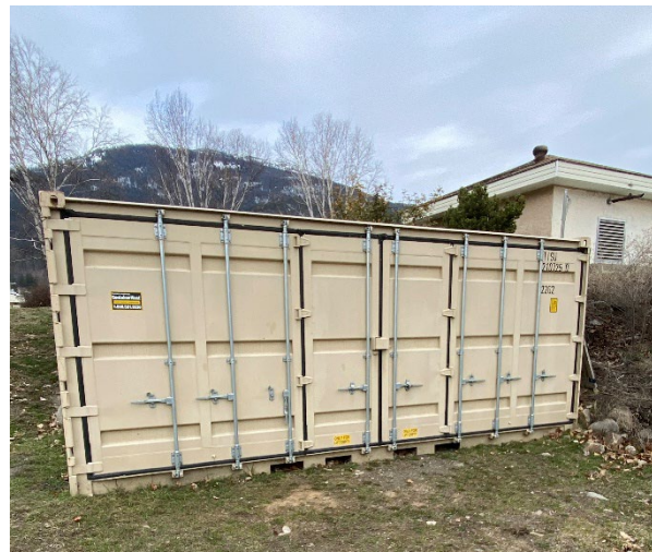
Sludge Dewatering Structure
