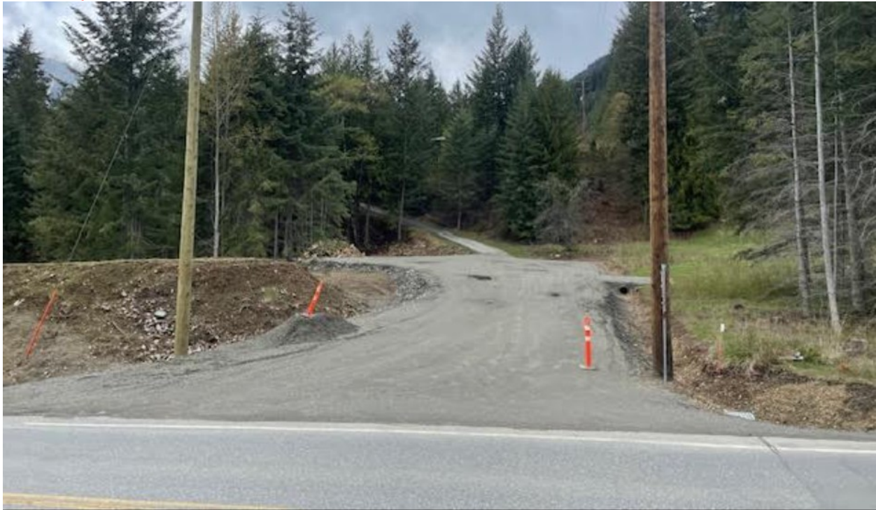
Boundary Ave with anchors removed and new pole and anchor installed
