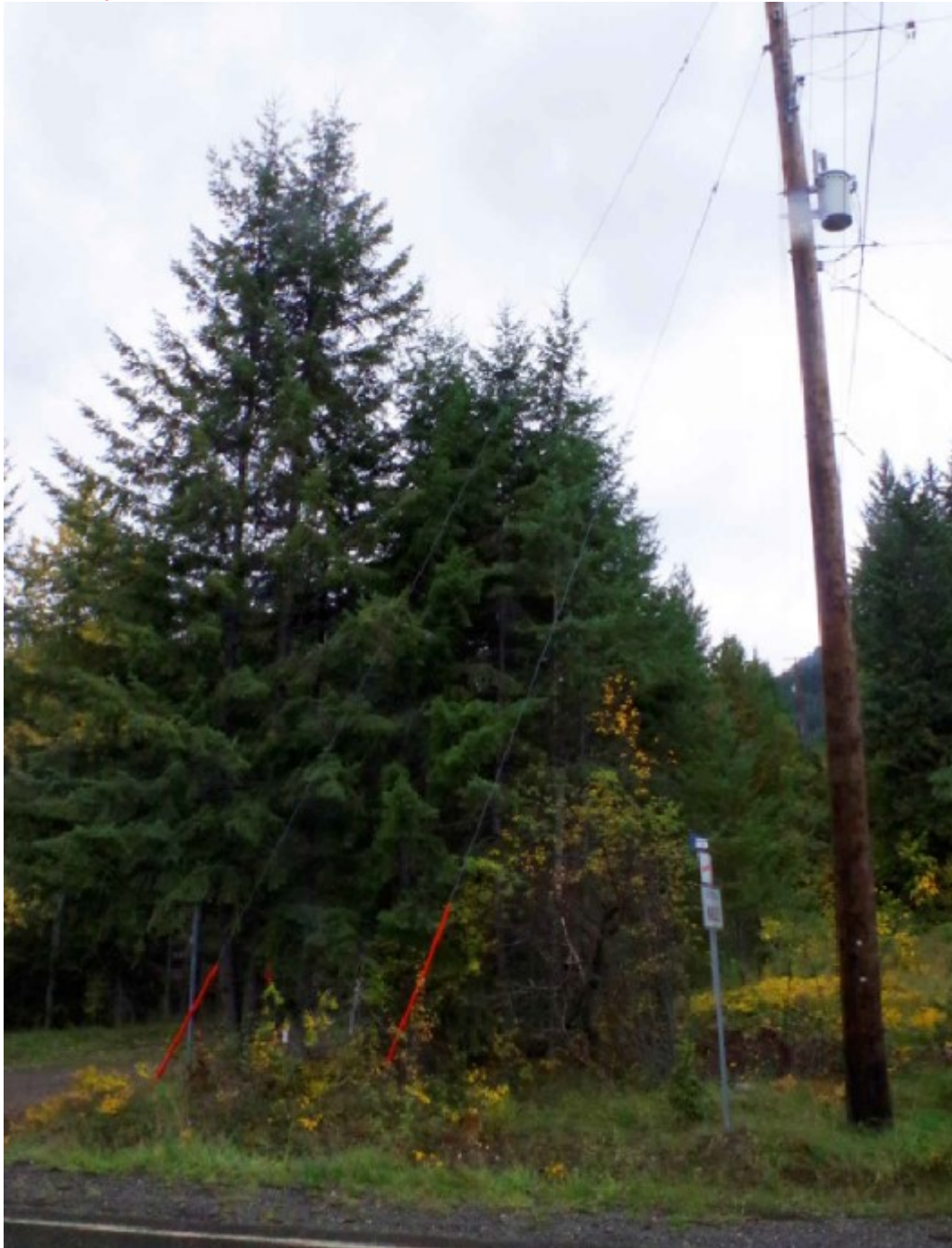
Boundary Ave prior to tree removal and road improvements
