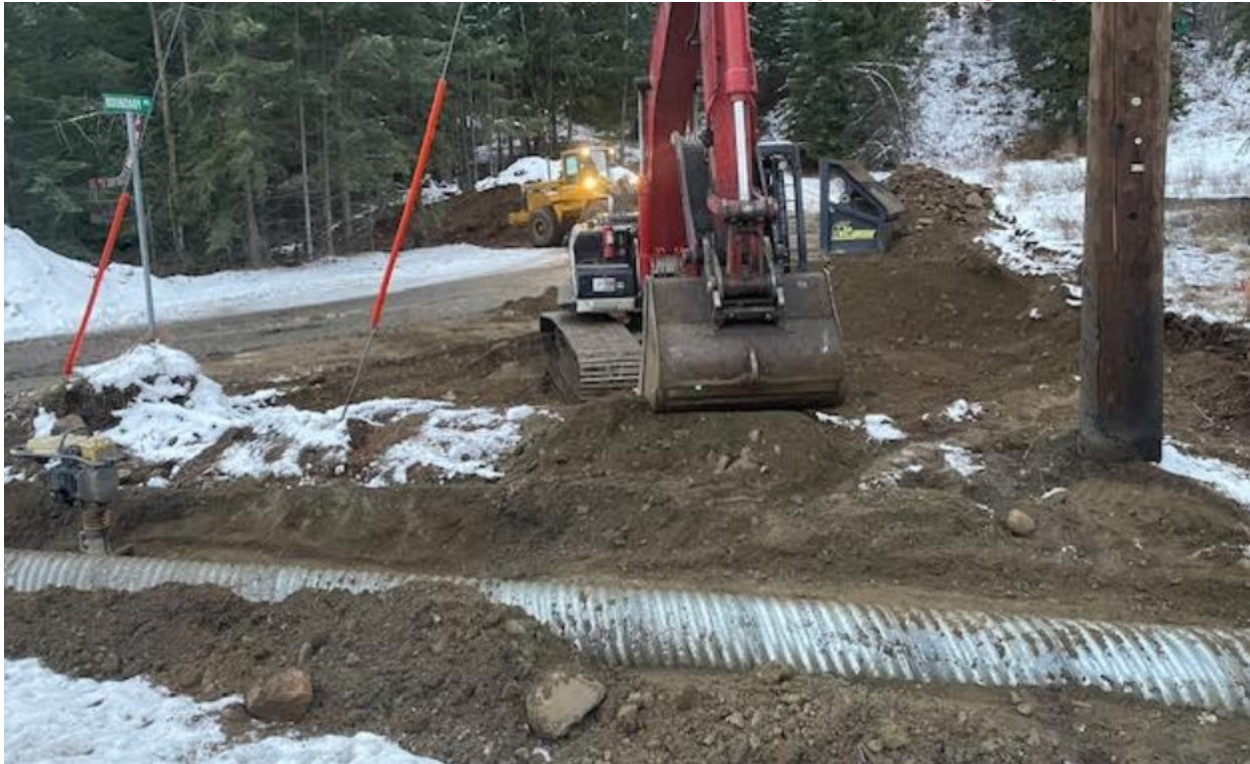
Installation of the 500mm culvert at the intersection of Boundary Ave and Highway 31
