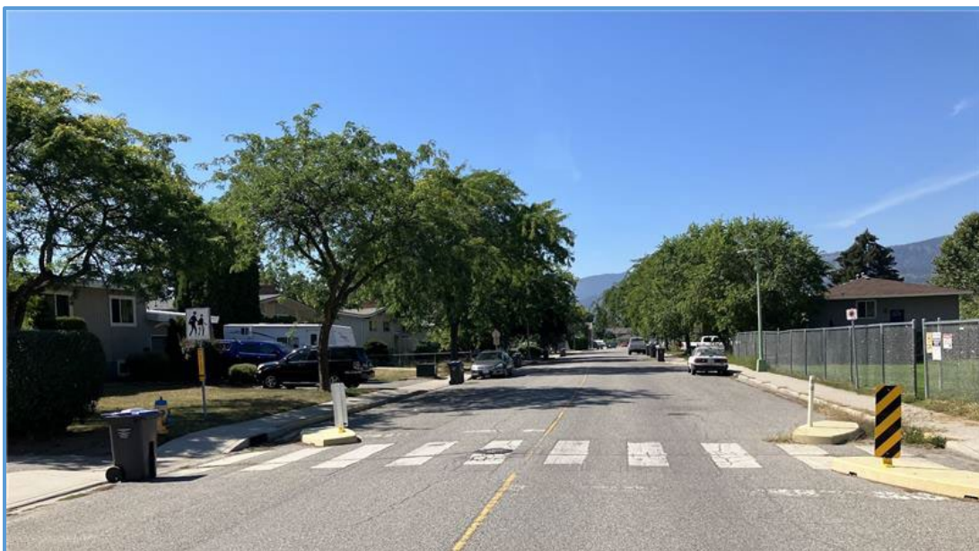
Figure 6: Midblock Crosswalk with Temporary Traffic Calming Curbs
